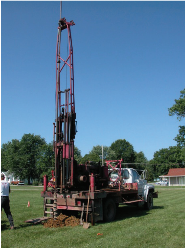
Auger Drilling Operation Figure 2-7
